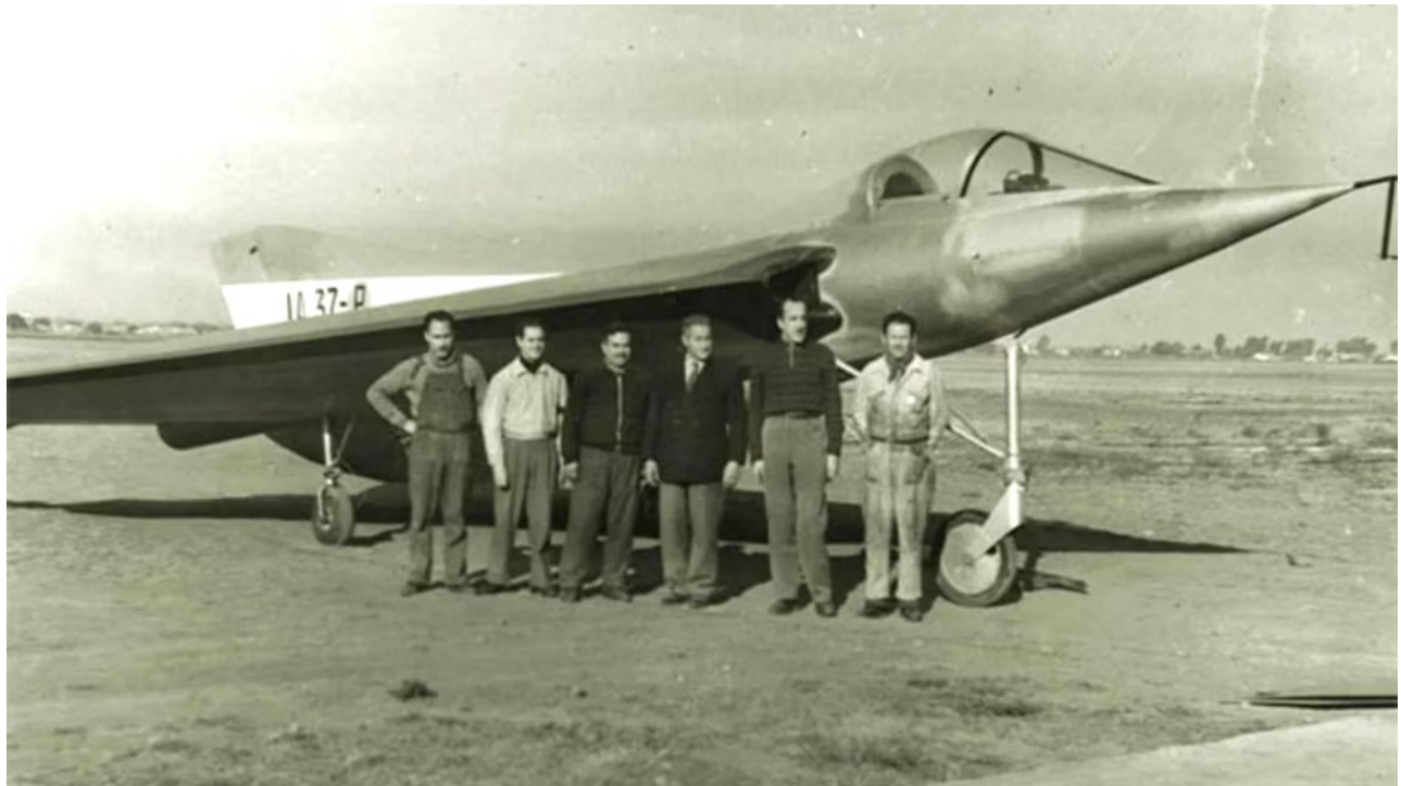
The IAe-37, a delta wing jet capable of Mach 2 speeds. (Photo: Via the author.)
